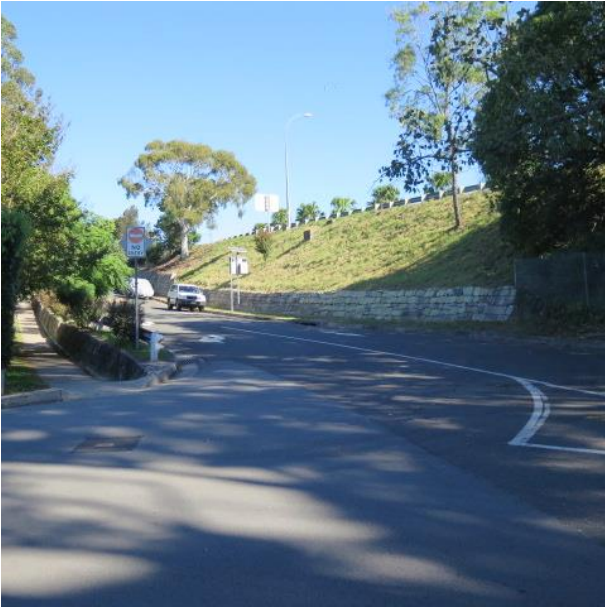
Figure 8 – View south in Reiby Street showing stone walls, heritage item I287, at foot of embankment of Burns Bay Road off-ramp.
