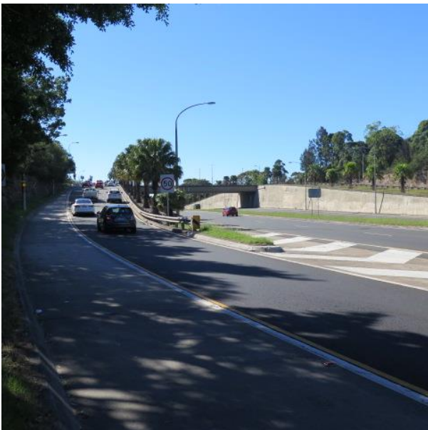
Figure 6 – Burns Bay Road off-ramp and overbridge from south.
