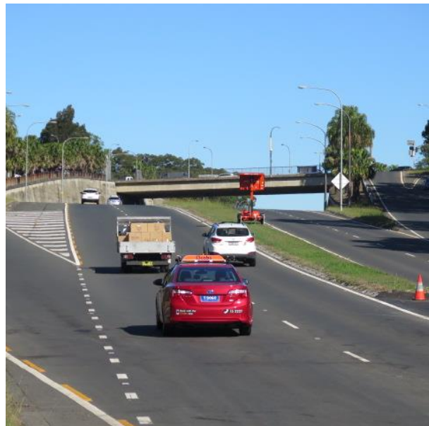
Figure 7 – Burns Bay Road off-ramp and overbridge from north.
