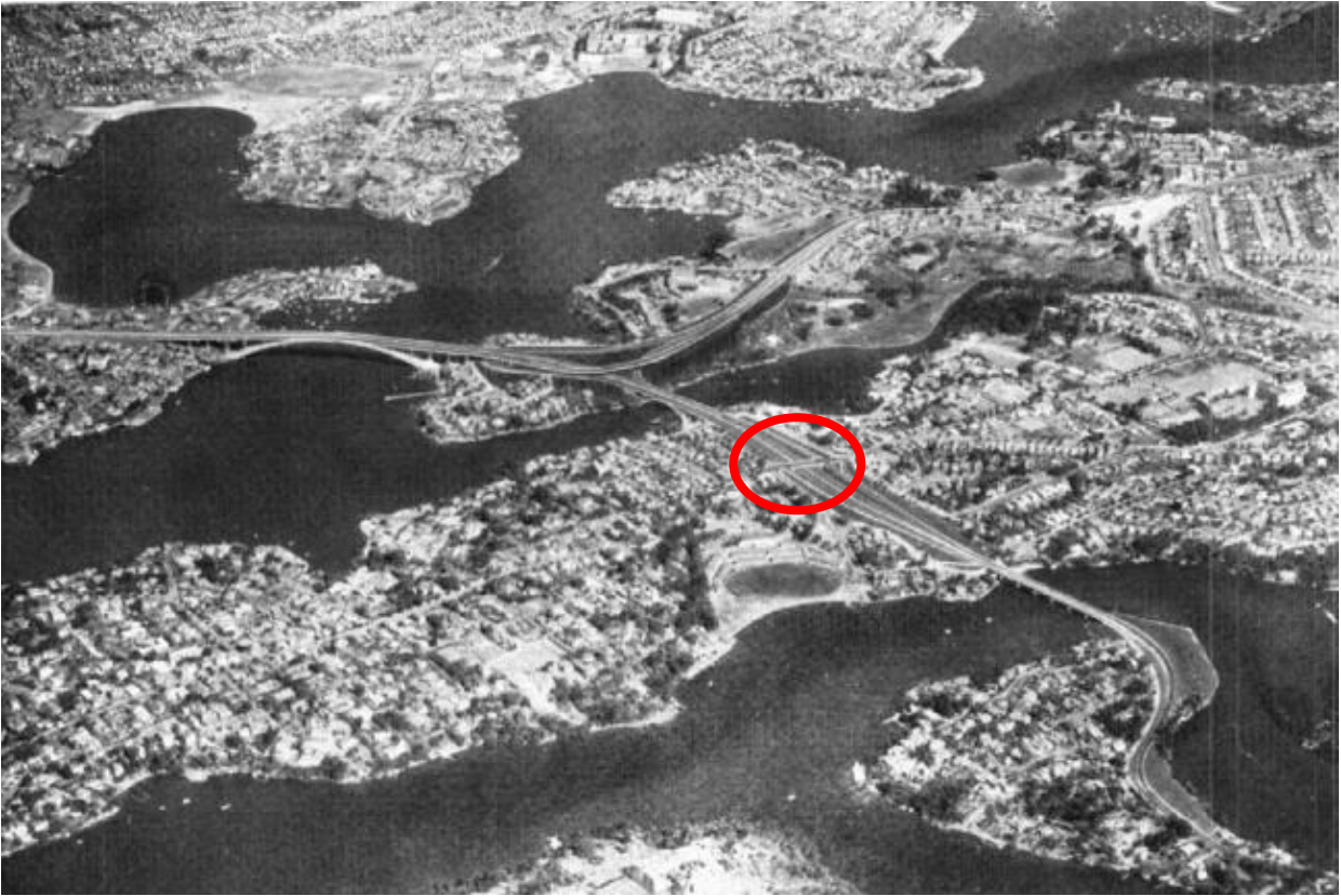
Figure 23 – “The North Western Expressway at Gladesville, Tarban Creek and Figtree Bridges. Tarban Creek Bridge, as completed, differs slightly in constructional detail from this artist’s impression”. Burns Bay Road Overbridge circled red.
